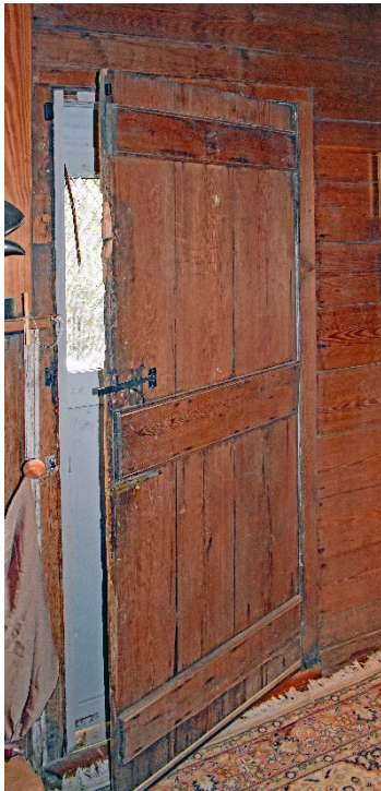
Figure 12. Batten door; south wall, south front room.
